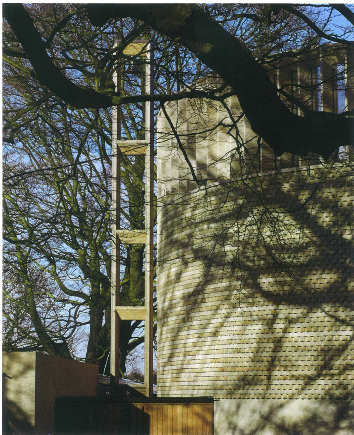
The bell tower rising above the entrance.
